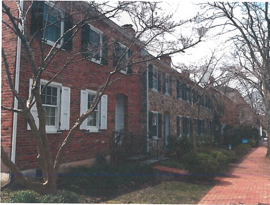
Figure 2. Row of 4 Townhouses on the site of the old Neisser school. 58E Wall St with brick façade is pictured in the foreground.
