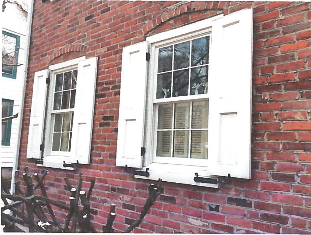
Figure 7. Anderson Woodwright Series 400 windows at 54 E Wall St – School St side of house
