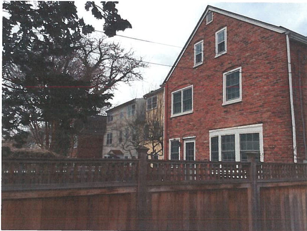
Figure 9. Recently installed Anderson Woodright Series 400 windows at 54 E Wall St – Rear of house
